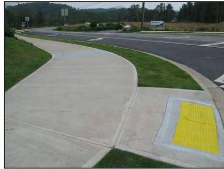
***A diagonal curb ramp with detectible warning.***
