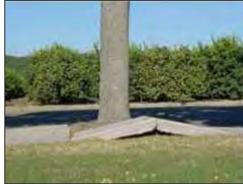
***Subsurface tree roots can lift concrete sidewalk slabs, causing the surface to become uneven.***
