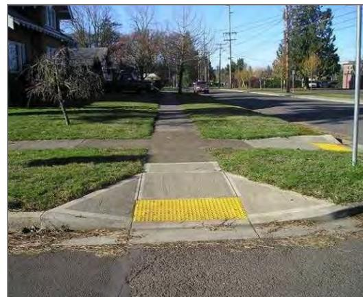
Example of an ADA-compliant perpendicular curb ramp
