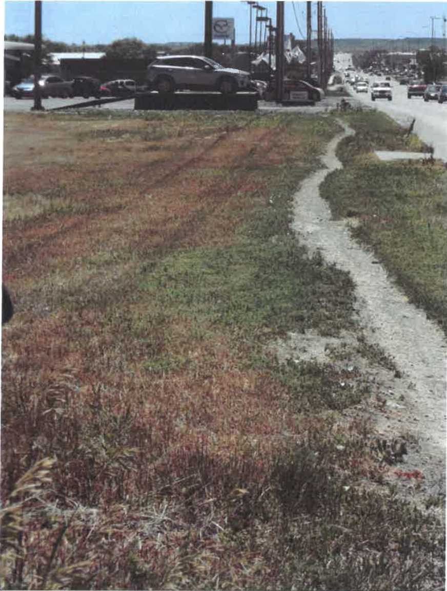
Cambell Street pathway from the start of the Mako Sica looking south toward Rapid Creek and the Leonard Swanson Pathway connection. Liberty Motors is on the left. A 10' sidewalk would need to be constructed along this section.
