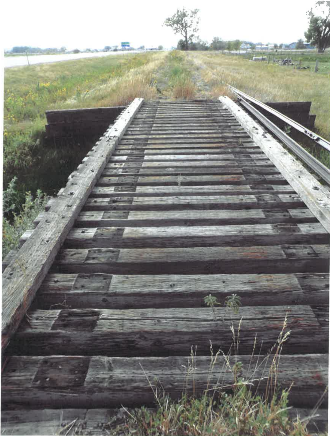
Railroad Corridor along Hwy 44 looking east
