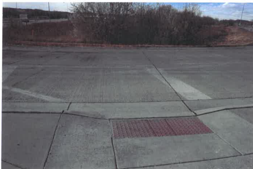
Curb Cut Adjacent to Trail
