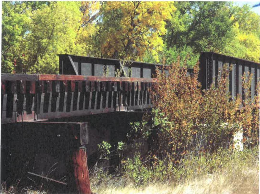
Rail corridor in Rapid Creek drainage with fall foliage.
