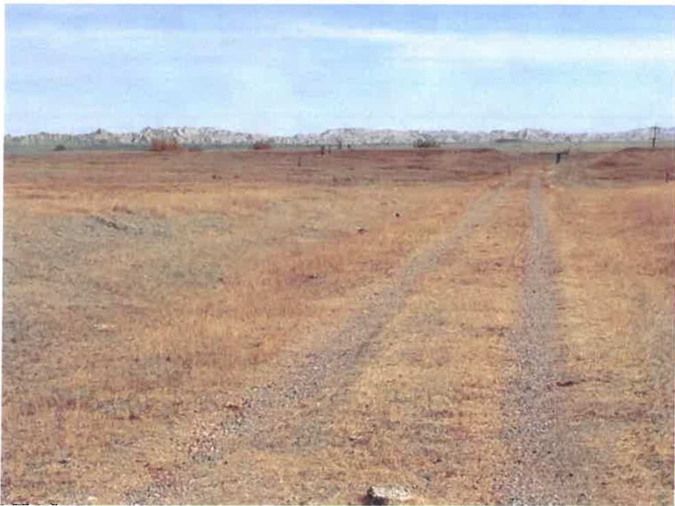
The trail corridor to Interior is suitable to be hiked or biked now if the bridges were decked.
