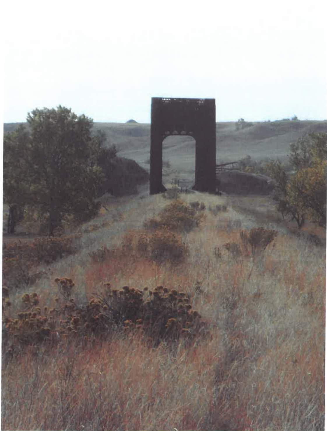
Cheyenne River Bridge standing as the gateway to the Badlands.
