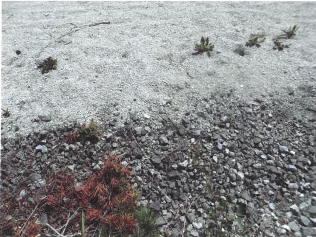
Crushed stone surface with a layer of limestone fines over the top
