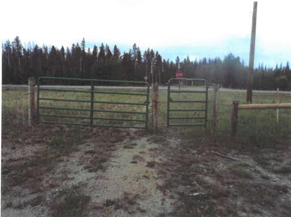
Gates for service & emergency vehicles as well as pedestrian, bike and equestrian
