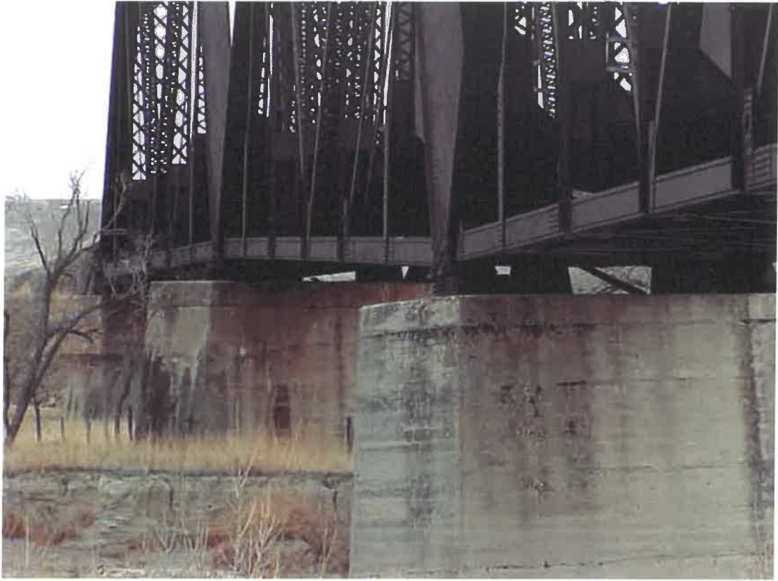
Cheyenne River Bridge before renovation
