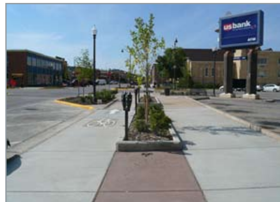
Bicycle track on Kansas City Street, Downtown Rapid City.
