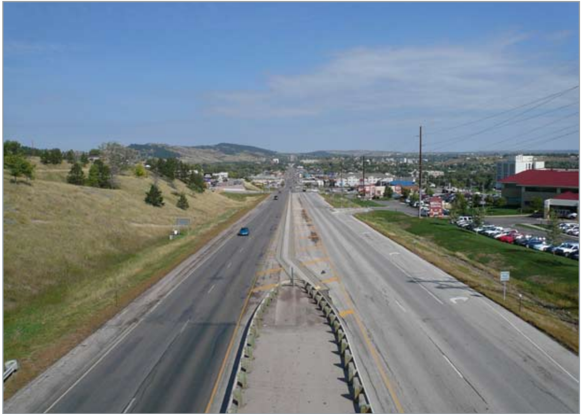
Above: Community Gateway. The median area at Tower Road and to the north is a prime candidate to accept gateway feature enhancements.
