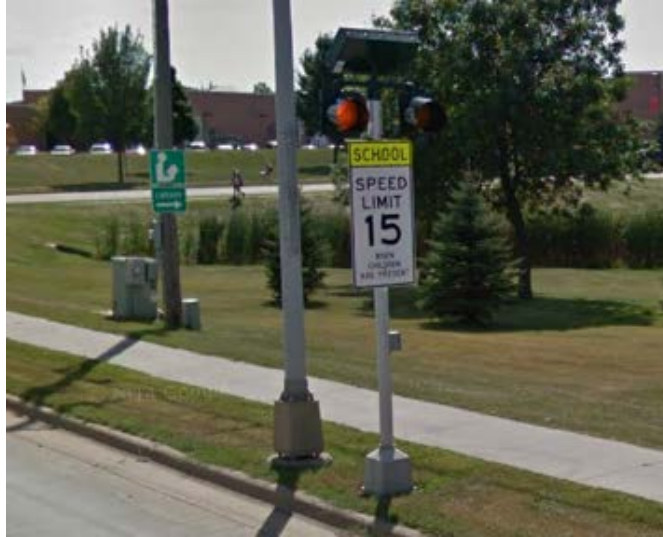
Figure 1 – School Speed Limit Sign Beacon installed near Washington High School on North Sycamore Avenue in Sioux Falls, SD
