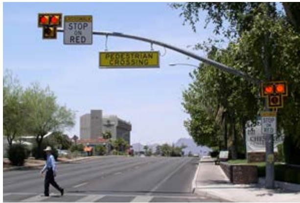
Figure 5 – Typical HAWK Installation
