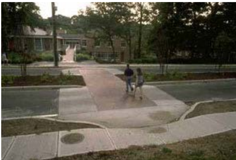
Figure 23 Raised pedestrian crosswalk or speed hump
